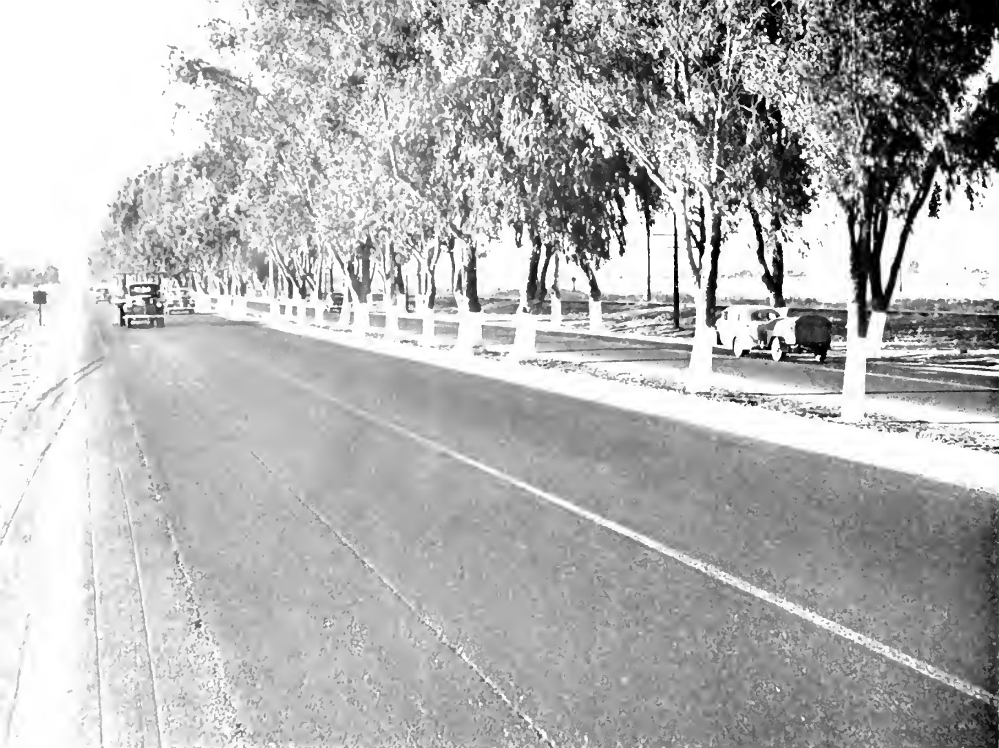
Newly completed divided highway south of Madera. Roadside trees of old road preserved as screen on division strip
